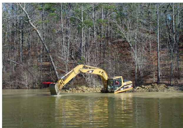
Heavy silt deposits should be removed with equipment to deepen lake edges.
